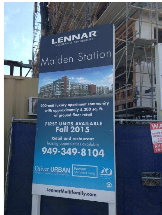
Figure 6. Malden Station Construction Site
