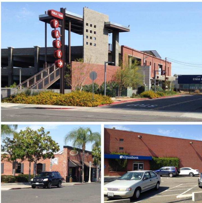
Figure 8. Red brick structures and accents on and near the study site
