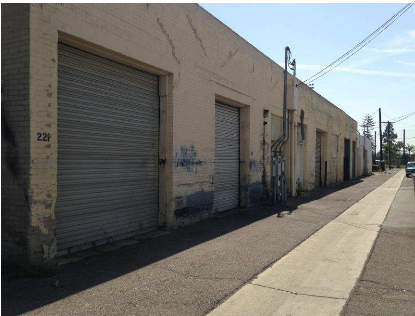
Figure 7. Rolling garage doors behind the Sanitary Laundry Building
