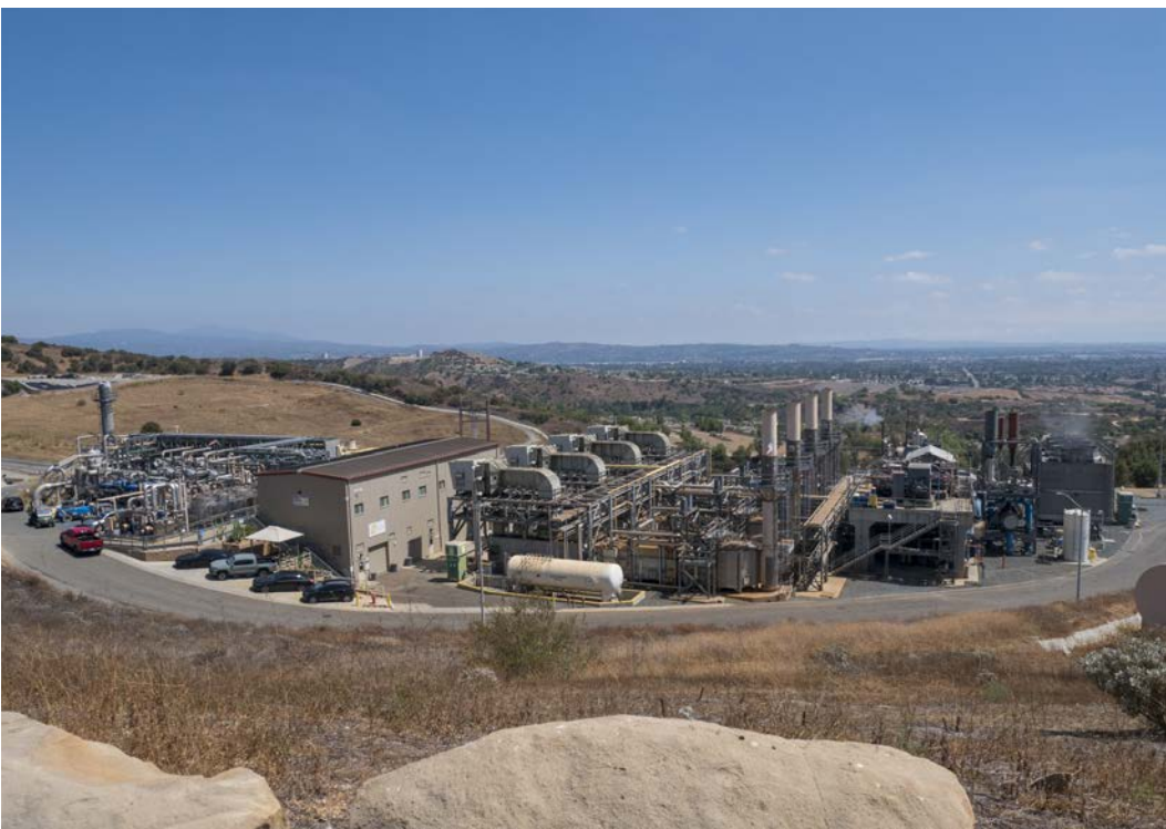
Left: George Hernandez, Deputy Director for Olinda Alpha Landfill, at the start of the landfill tour showing where trash is placed each day before being compacted and covered with a layer of soil or tarps. Right: Third-largest landfill gas-fueled plant in the U.S. at Olinda Alpha Landfill - converts landfill gas to energy which powers over 36,000 average Orange County homes. PHOTOS COURTESY OF EMMERSON LITTLE
