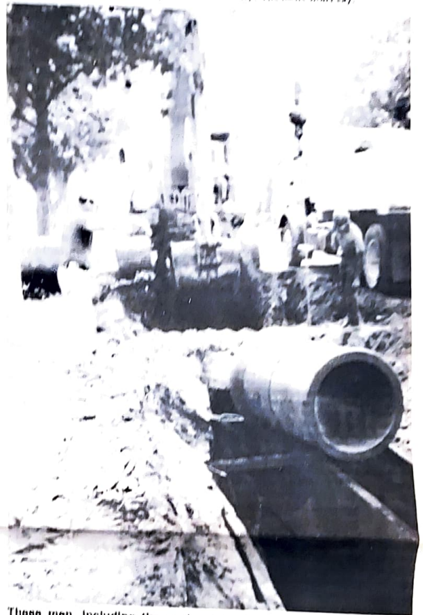
These men, including the worker barely visible in this underground sewer trunk on Malvern Avenue, are working to complete the major overhaul of Fullerton's sewer system which has been winding its way through the heart of the city for the last 4 months.
