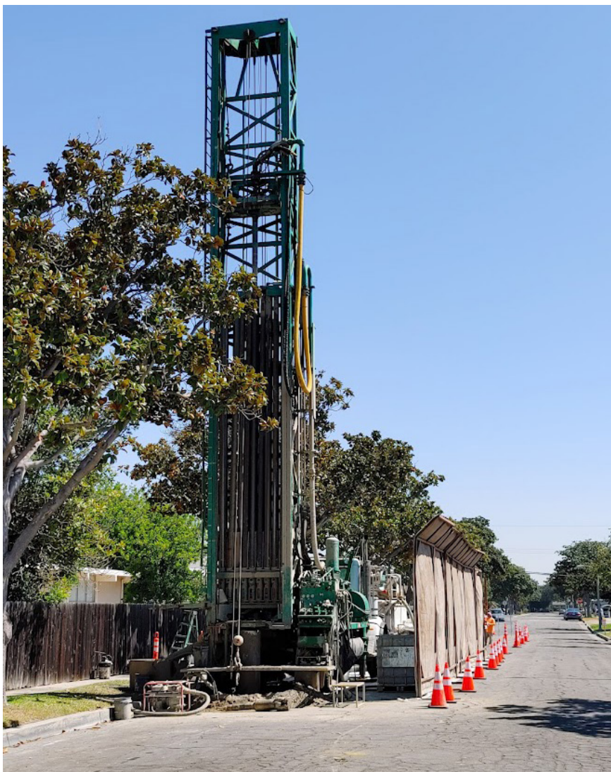
Drilling and well installation at the Orange County North Basin Superfund site.
